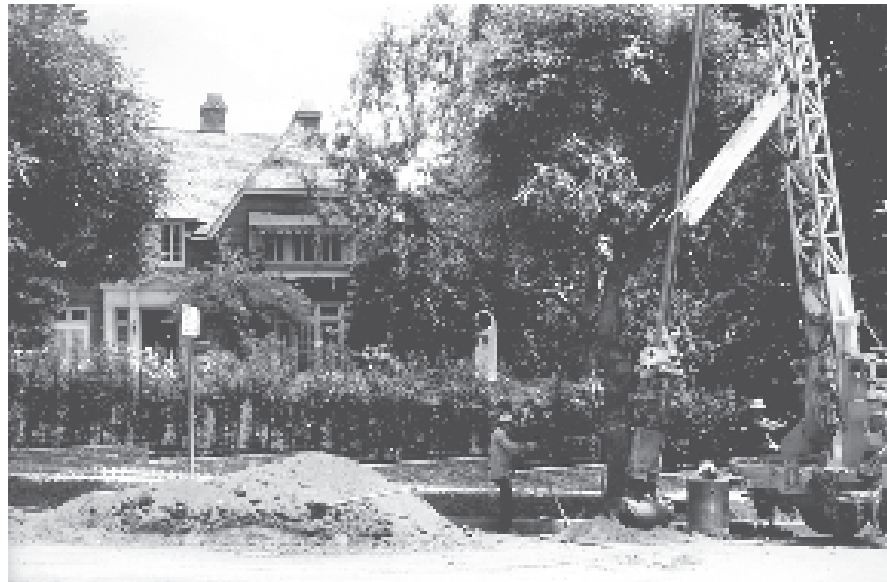
The Hollywood Trench
