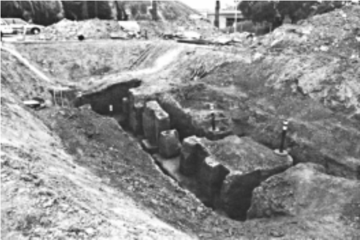
Figure 7. Southward view of hand-excavated trenches dug into base of the large rectangular excavation, which approximately coincides with the base of artificial fill. Faults strike from upper left to lower right corner of photograph. Note cars in upper left corner for scale.
